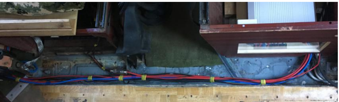
In between some cables:
